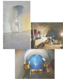
FIG. 2: Some photos in the KAGRA facility. Top Left: spiral stairs from the ground level to the upper level for the suspension tower. Top Right: installation of the granite stone for the geophysics interferometer. Bottom: transportation of the cryostat to the end room.
